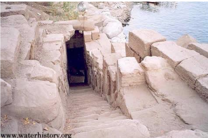
Figure 2.4 : The nilometer on Elephantine Island, Aswan, consists of stairs and staff gauges. Source: [27]
